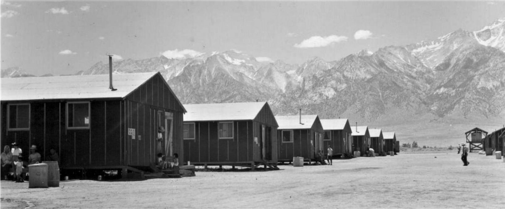
Barracks of Manzanar Internment Center, Sierra Nevada Mountains beyond, Owens Valley, California, 2 July, 1942 – Author, Dorothea Lange, U.S. National Archives, Wikimedia. Uninsulated barracks in the desert were ferociously hot in summer, freezing in winter.
