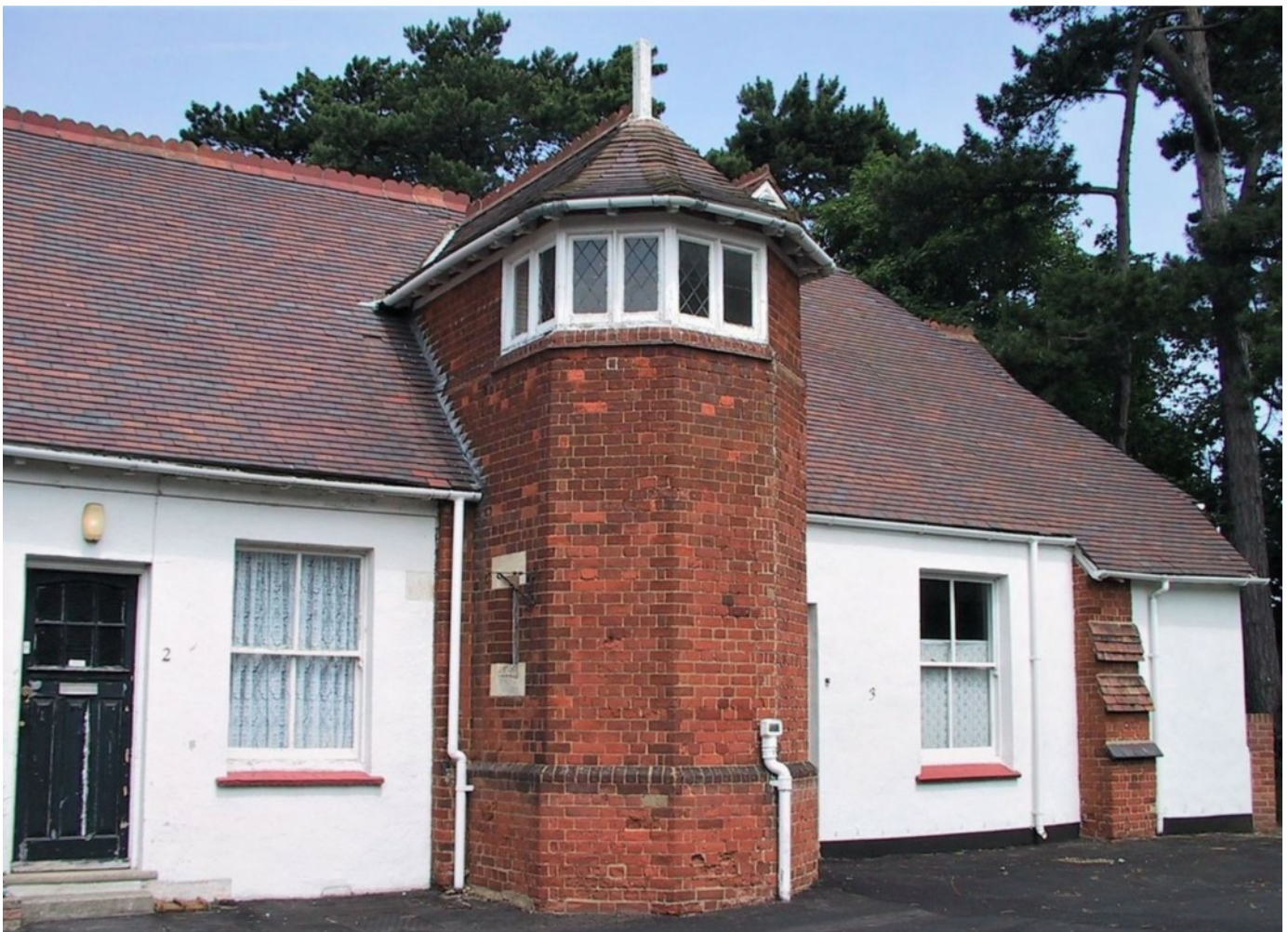
Cottage at Bletchley Park , formerly a tack and feed house where Alan Turing worked in 1939 and 1940 developing the electromechanical machine Bombe that broke the German naval Enigma military code – Author, Matt Whitby, Public domain, Wikimedia
